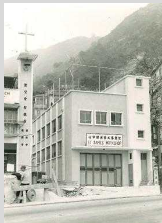
聖雅各工藝訓練中心 St James' settlement workshop Building
